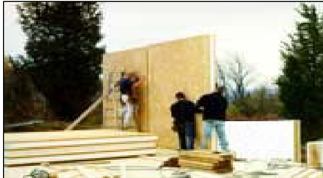
Figure 11- Structural Insulated Panels (SIP)
