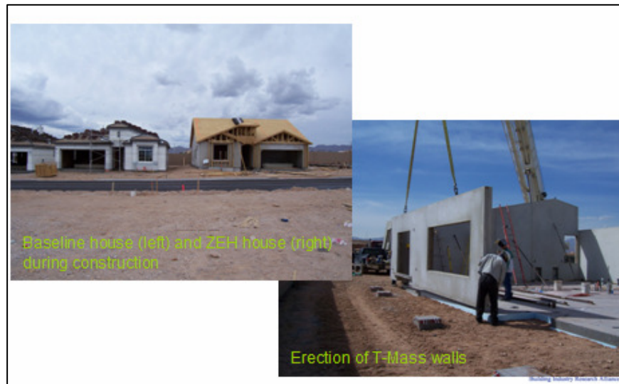
Figure 23- Construction at Vinings, Las Vegas
